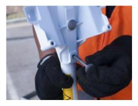
Use Carriage bolts, and Serrated Flange Hex Nuts.
