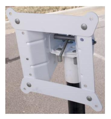
Install the AZ/EL Mount Assembly onto the mast pipe. It may be necessary to loosen the three bolts on the canister to allow the assembly to slide over the mast pipe.
