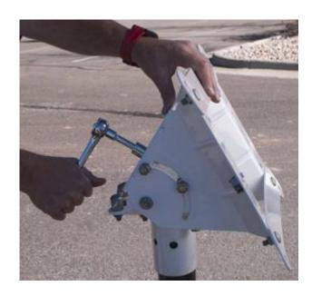
Do not lockdown the elevation bolts until finished with adjusting the elevation.
