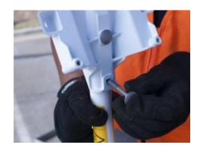
Use Carriage bolts, and Serrated Flange Hex Nuts.
