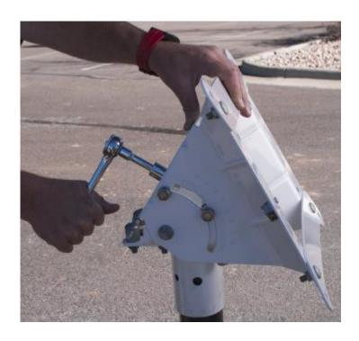
All four elevation lock down bolts need to be loosened and their four associated lock washers disengaged prior to beginning the adjustment of the elevation process.
