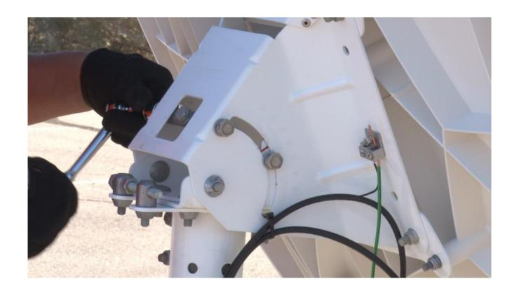
Use the wrench on the Elevation rod nut to adjust the elevation up or down.
