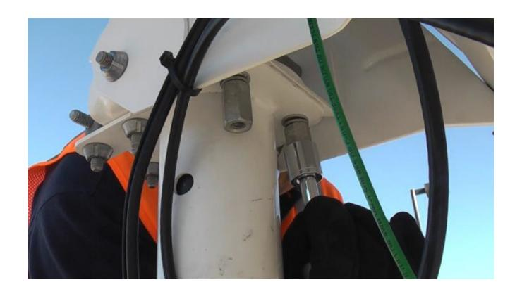
Using a wrench, rotate the hex head of the Azimuth fineadjust bolt.
