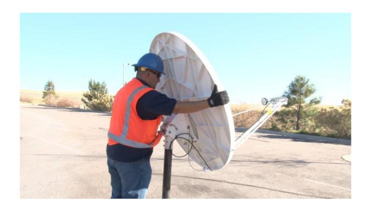
From behind the antenna, gently push and pull each side of the antenna.
