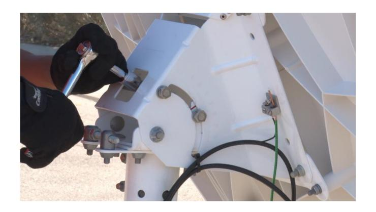
Slightly loosen the 4 Lockdown Nuts in the Arched Slots on sides of the Elevation Bracket
