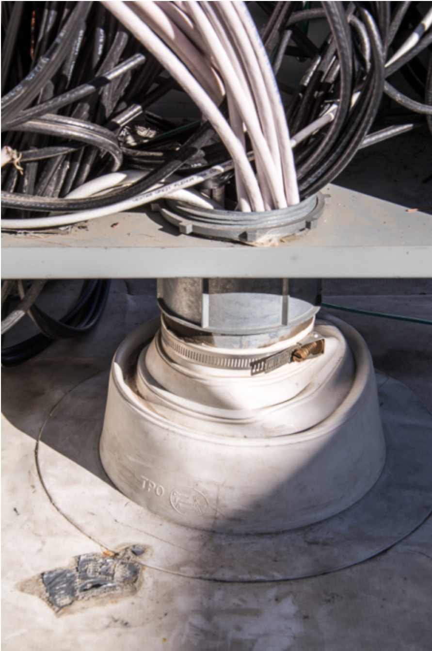
Roof Flashing
