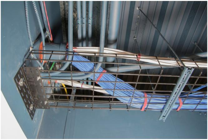
Important! Always use the proper cable support system in a building. This ensures the customer has the best installation
