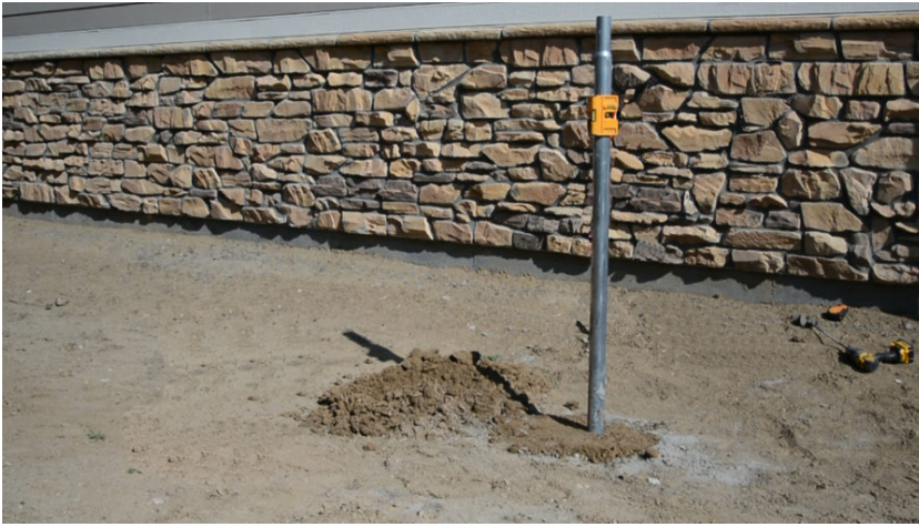
Pole Mount Job Aid – Concrete Mix
